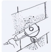
Preparation of the cut for the semi-cylindrical and circular segment flat jacks using a cutting saw
